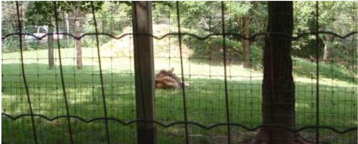
FIGURE 4.8 This lion enclosure at The Killman Zoo is an example of a lion enclosure constructed of deer fence and a lower secondary layer of wire mesh.
